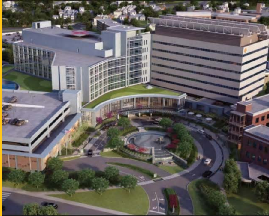
Danbury Hospital, Danbury, CT
